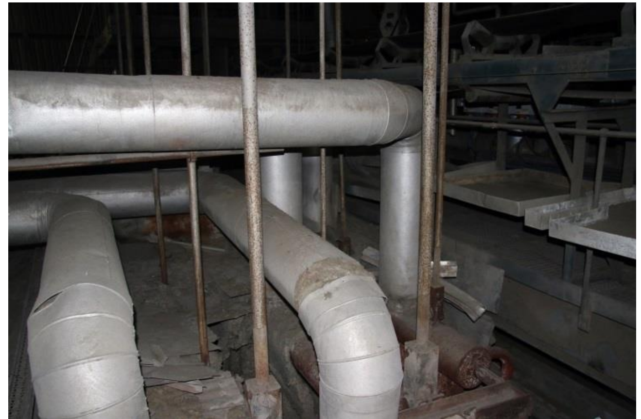
Hanger Rods – Bottom Connection Details
