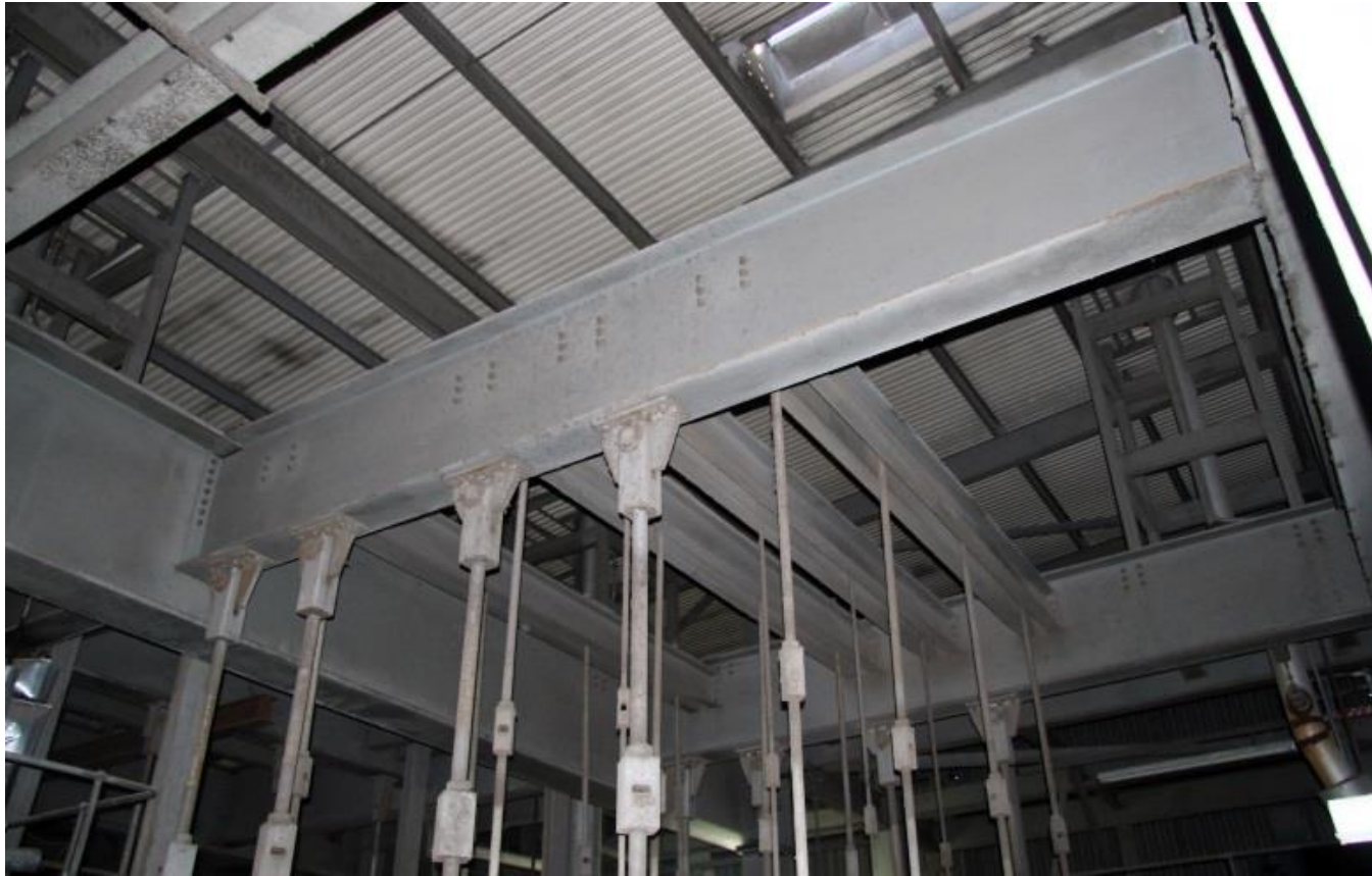
Hanger Rods – Top Connection Details
